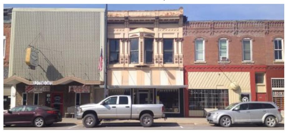
Two to three stories 2,000 – 5,000 sq. ft. Masonry bearing wall structure
